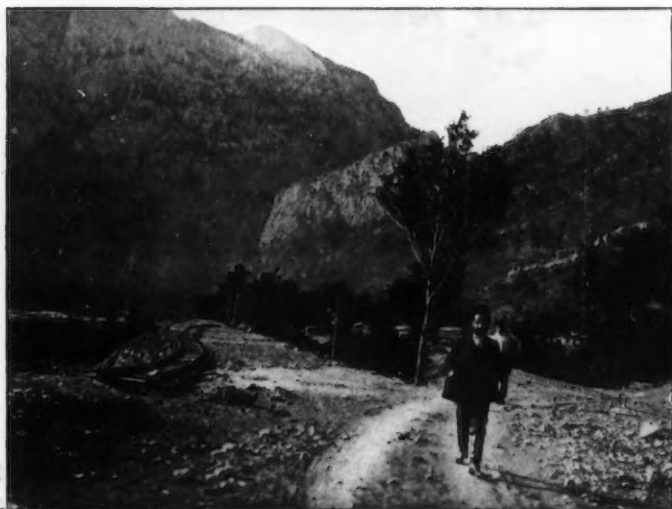
KARAPUNAR VILLAGE AND NORTH END OF FIRST TUNNEL, TAKEN FROM 1 KILOMETRE BEYOND KARAPUNAR.
